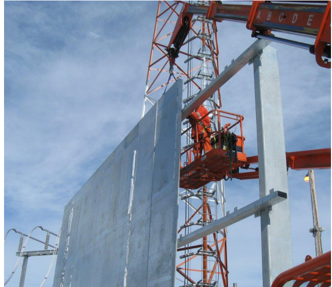
Acoustic DuraBarrier being installed next to loud machinery.
