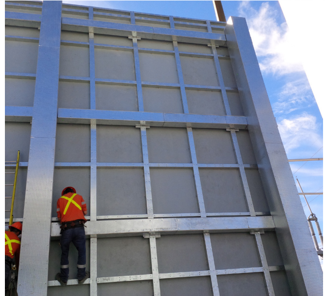
A Ballistic DuraBarrier installation with girt protection.
