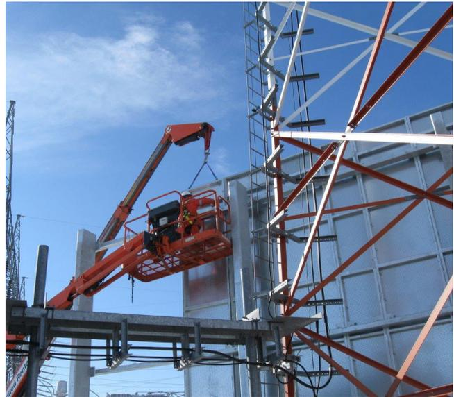
DuraBarrier module being installed.
