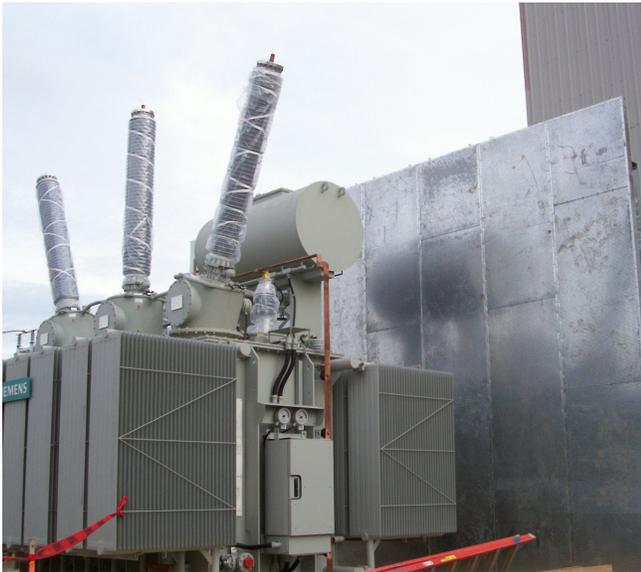
The front face of a DuraBarrier Installation.
