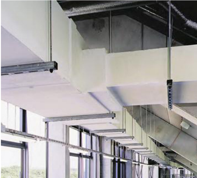
DuraDuct 3HR installation.
