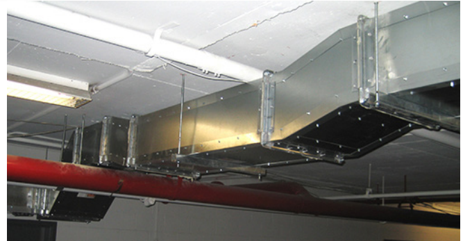
DuraDuct GNX installation in an underground parking garage.
