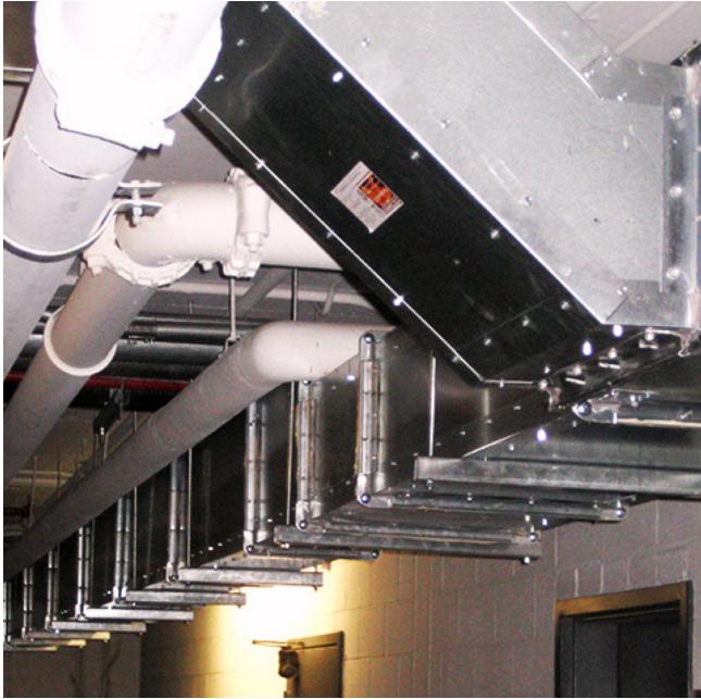
DuraDuct GNX installation in an underground parking garage.
