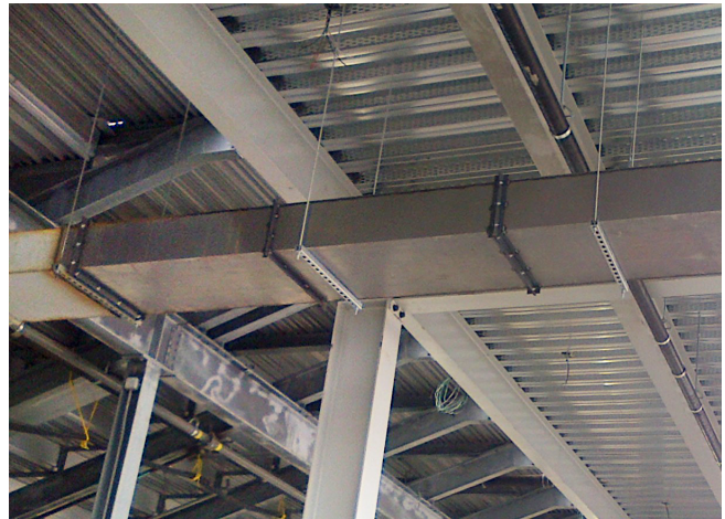
DuraDuct SED connected to an existing exhaust system.
