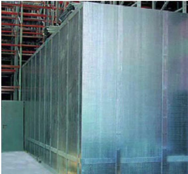
An Acoustic Enclosure.
