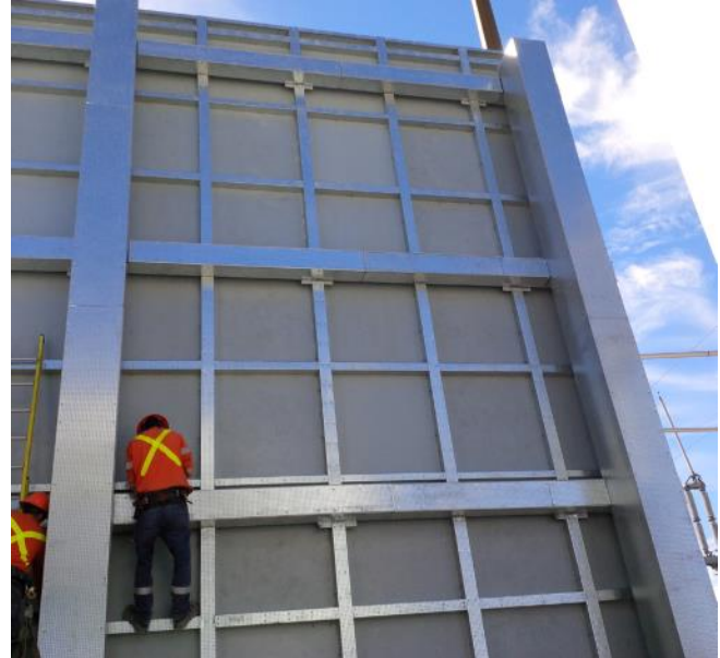
A Ballistic DuraBarrier® installation with girt protection.
