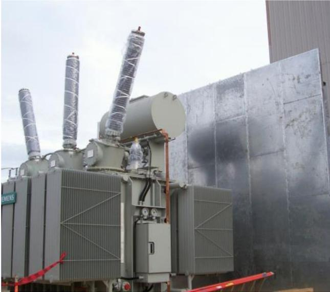
The front face of a DuraBarrier® Installation.
