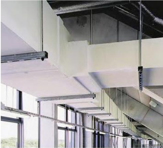
DuraDuct™ 3HR installation.
