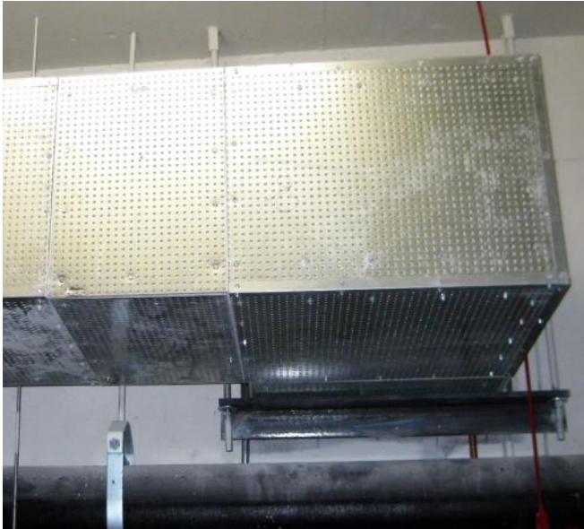
DuraDuct™ 4HR installation.
