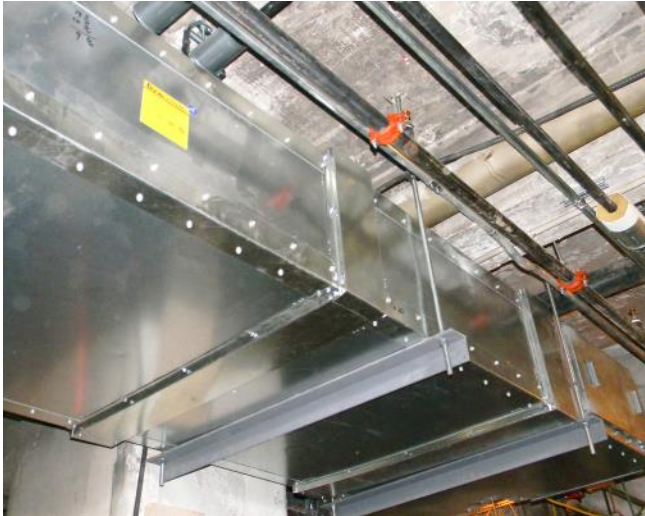
DuraDuct™ KEX Installation.
