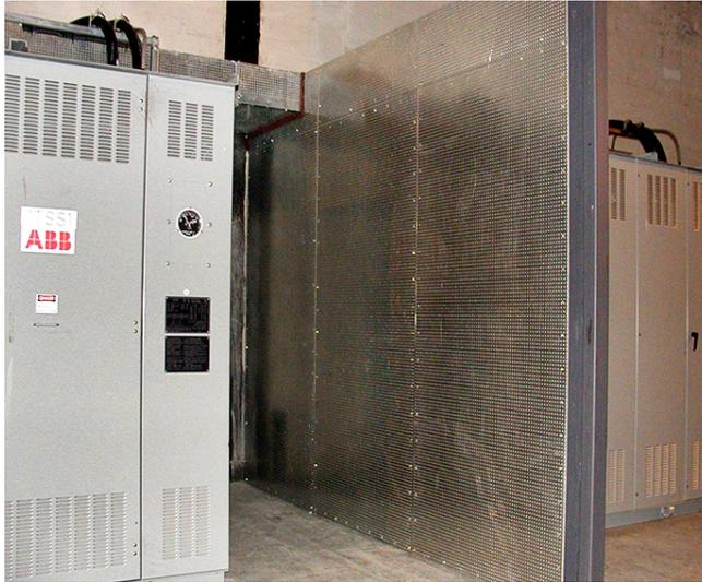
A fire wall separating two electrical enclosures.
