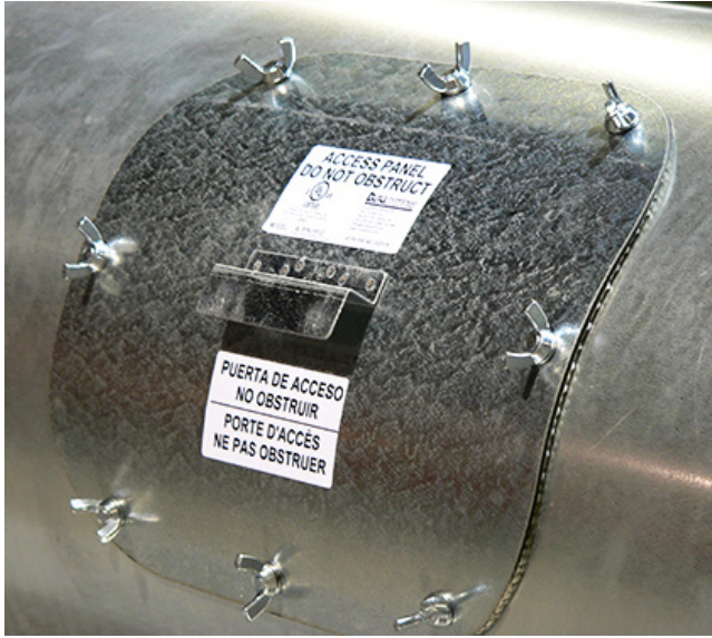
A curved access door installation.
