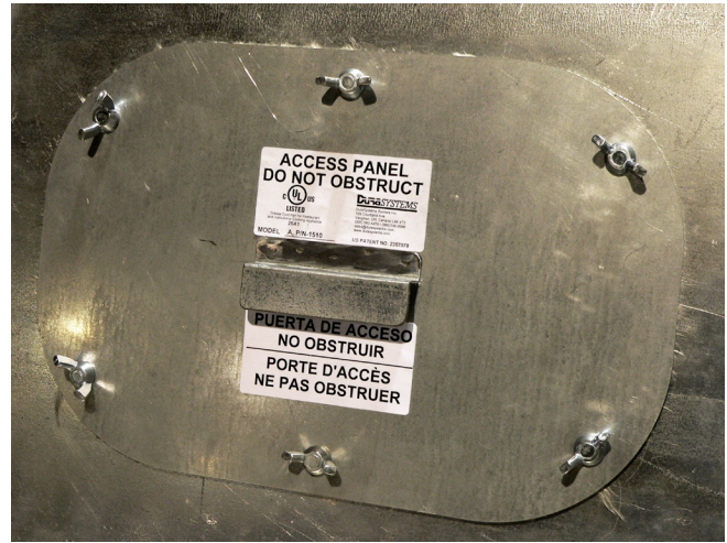
A flat access door installation.
