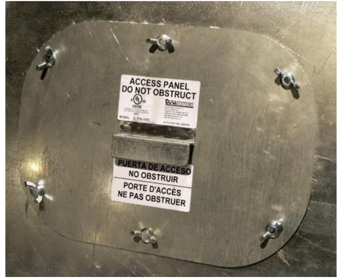
A flat access door installation.
