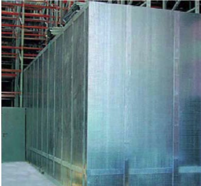
An Acoustic Enclosure.
