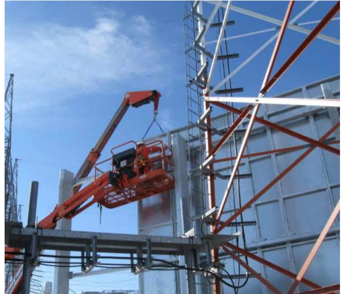
DuraBarrier® module being installed.
